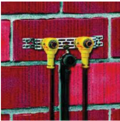
Wash basin installation: Everything fitted to the exact dimensions.
