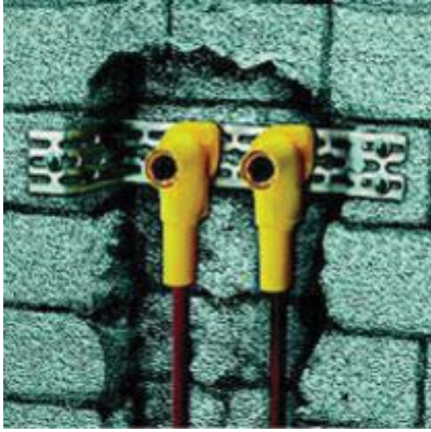
Wash basin installation: Installation in tight wall recesses
